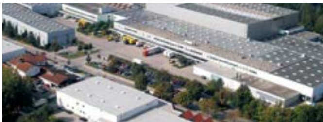
Häfele Distribution Centre Nagold, Germany
