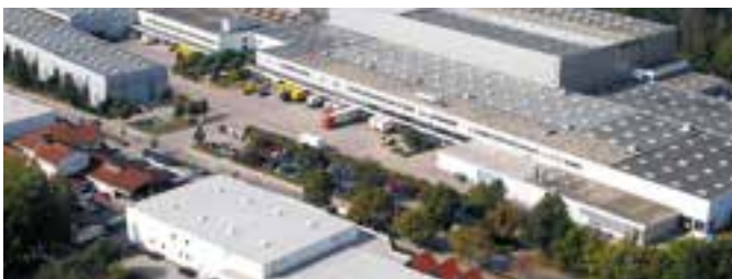
Häfele Distribution Centre Nagold, Germany
